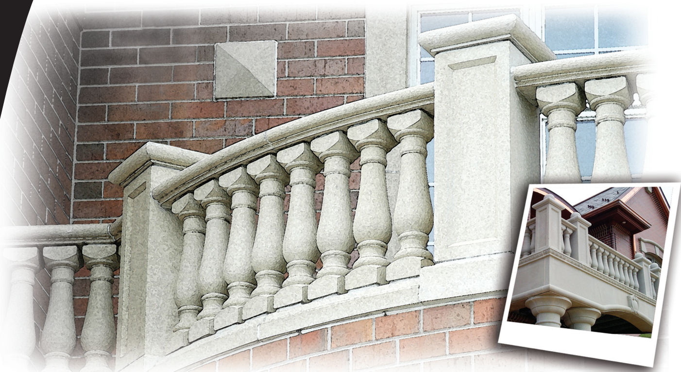
Plain view of top rail and piers.
